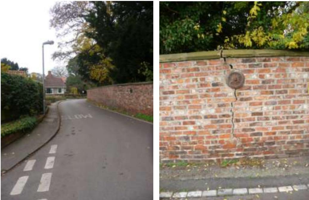
*Plate 6. The listed wall which forms the boundary to Butts Lane. It already presents structural cracks and leans slightly towards the road. There is no buffer to protect it from damage caused by heavy vehicles.*
